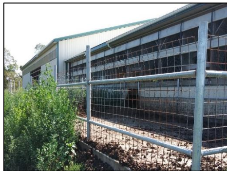
BEFORE: congregation area with uncontained manure. AFTER: One of two roofed heavy use areas (HUA) to contain manure and separate stormwater from animals and manure. The two HUAs replaced the metal fenced area in before photo.
