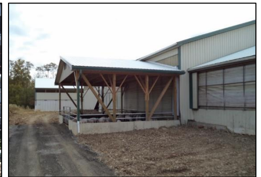
BEFORE: congregation area with uncontained manure. AFTER: One of two roofed heavy use areas (HUA) to contain manure and separate stormwater from animals and manure. The two HUAs replaced the metal fenced area in before photo.
