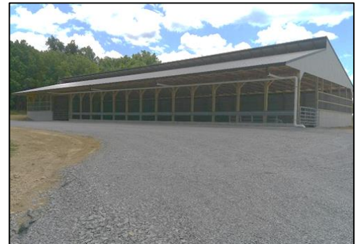
BEFORE: Brown congregation feeding lot with uncontained sediment and manure. AFTER: Completed heavy use area (HUA) and waste storage facility with roof.
